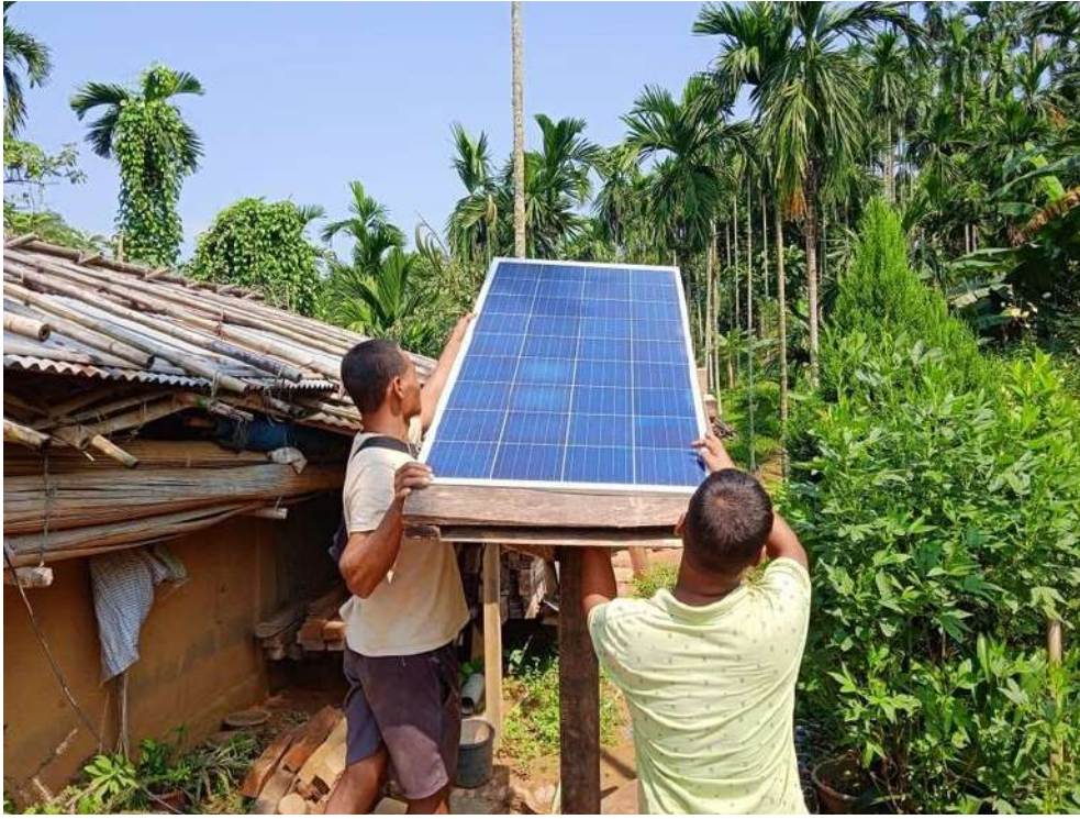
Fig- Installation of Solar Microgrid in Chokpot block, South Garo Hills
